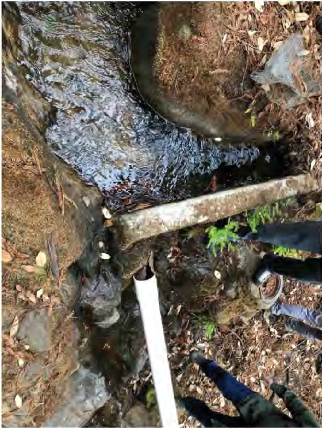
Repaired South Creek raw water intake
