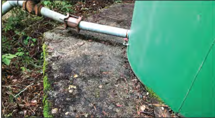
Figure 12: Oberst Station existing foundation
