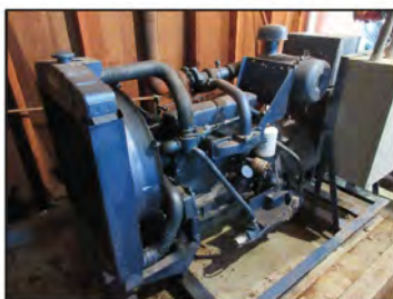
Figure 9. Generator repaired and operational
