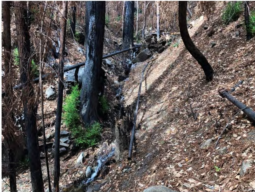
Corvin Creek intake not yet repaired.
