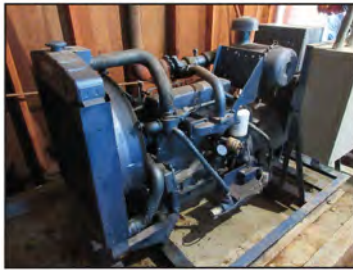
Figure 9. Generator repaired and operational
